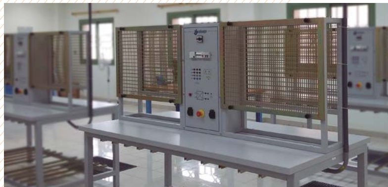
Electrical Installation Laboratory. COE MUHAYIL – ARABIA SAUDI
